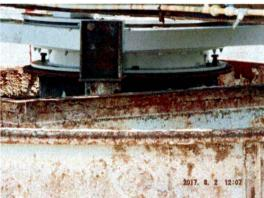
The Torque Cage and Adaptor Pads are in need of scraping, re-welding in some areas, sandblasting and coating with Coal Tar Epoxy
